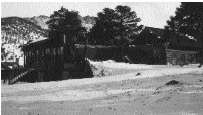
Collapsed Dining Hall, spring 1913.
