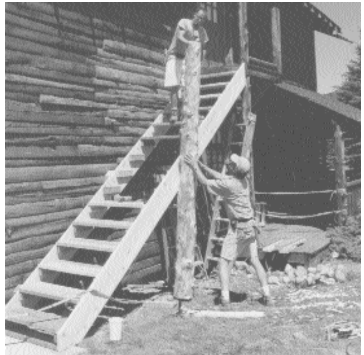
Buildings & Grounds rebuilds the fire escape.
